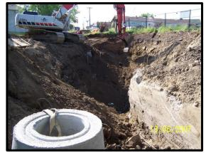
Image C-1: Manhole Replacement (June 19, 2007; Facing Southeast)
