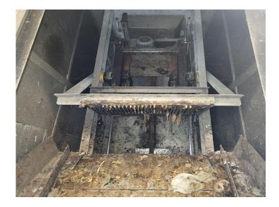
> The grating is broken and needs to be replaced.
