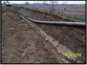
Image B-2: Forcemain Installation – During Construction (December 13, 2006; Facing Northwest)
