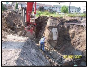
Image C-2: Manhole Replacement (June 19, 2007; Facing Southeast)
