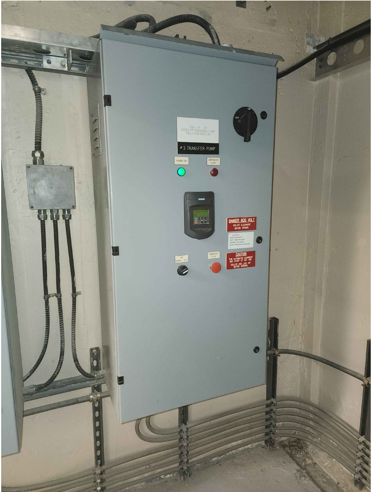
P1 EXISTING FILTER TRANSFER PUMP 2 & FILTER TRANSFER PUMP 3 E101 SCALE: N.T.S.
