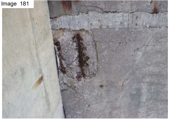
Girder 5 south end spall
