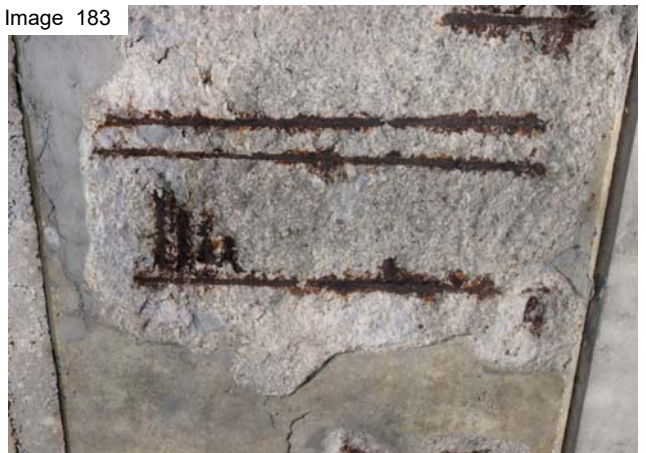
Girder 5 south end spall
